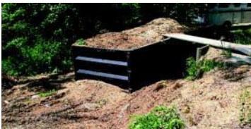
Before working with the Watershed Agricultural Council, this farm’s manure container provided a hard-to-access and dangerous set-up which resulted in unsanitary waste disposal that potentially threatened water quality.
